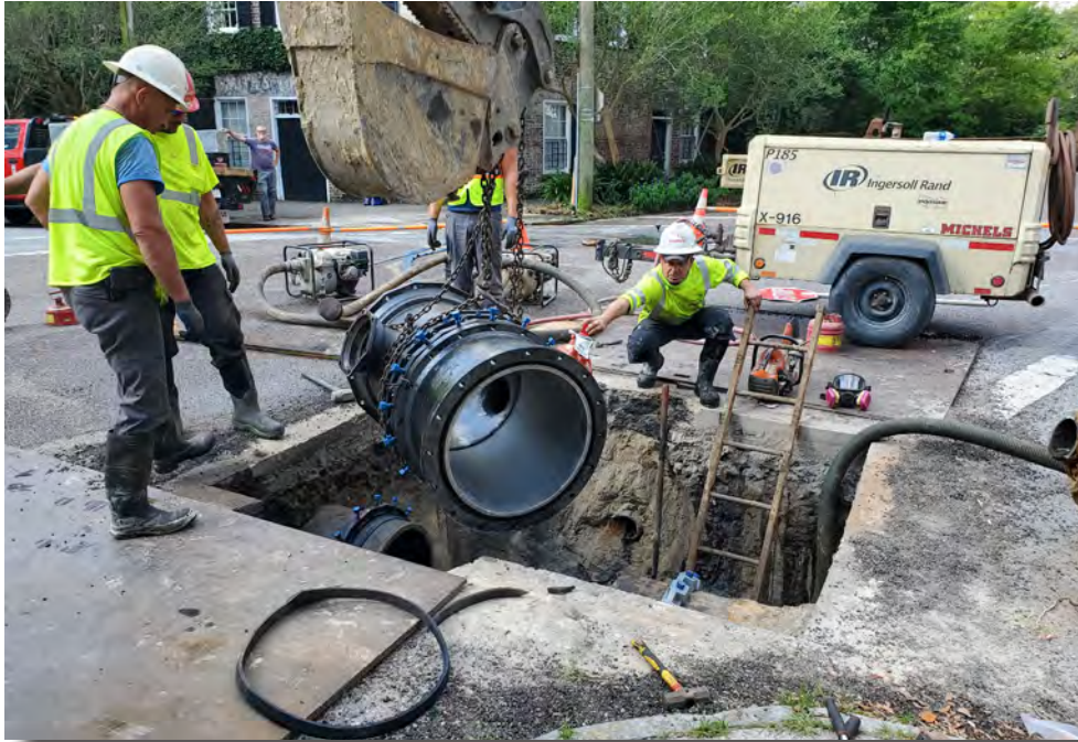
Peninsula Water Main Rehabilitation Phase 3
