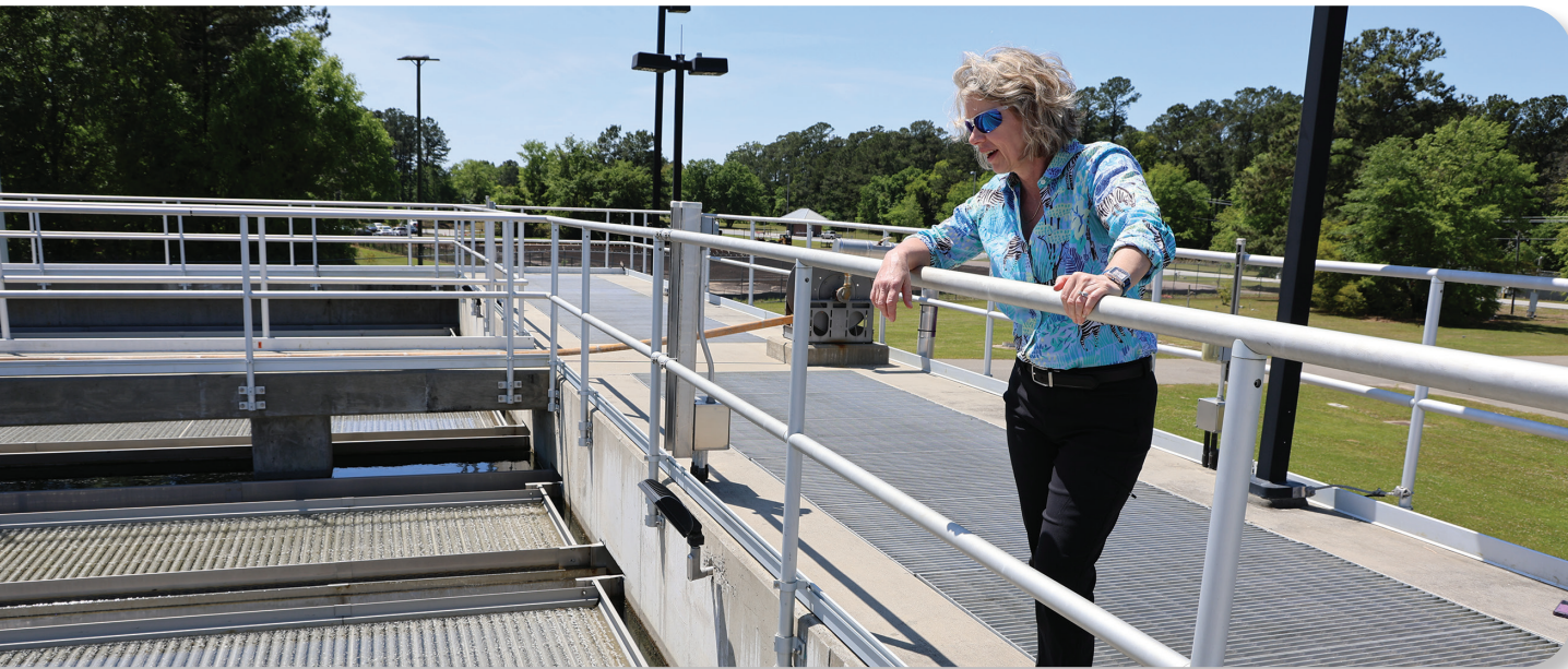
Director of Water Treatment Dr. Jane Byrne inspects plate settlers, which help to remove clumps of particles near the beginning of our water treatment process.
