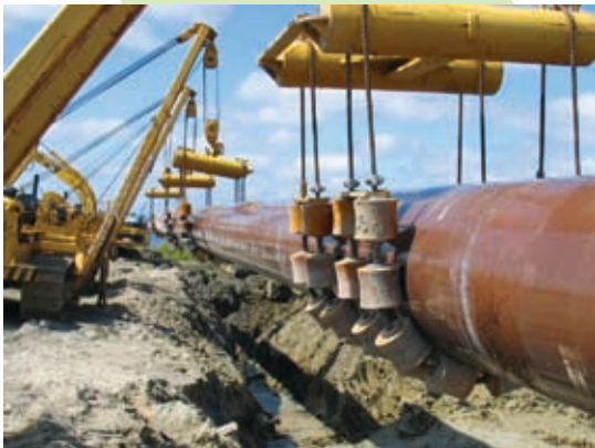
Construction of the new 40-inch water main under the Cooper River, which now serves the East Cooper area.
