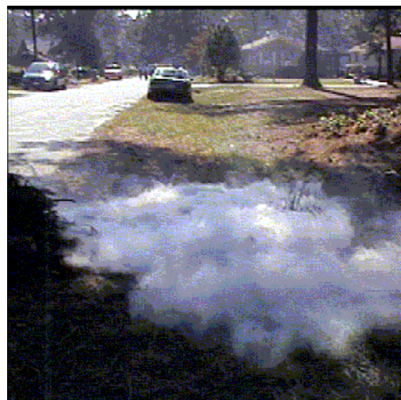
Figure 2. Smoke-testing on the wastewater collection system
