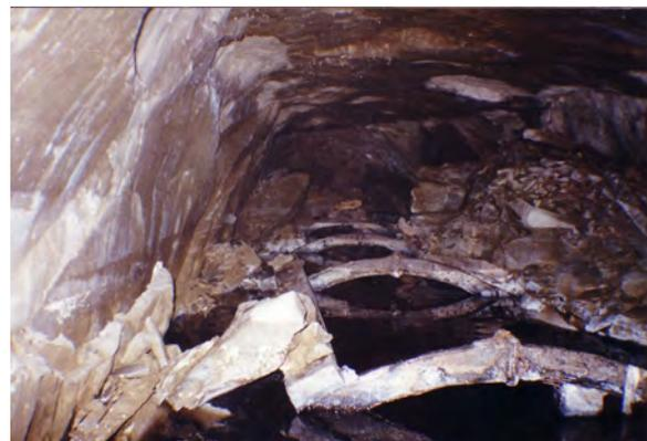
*This photo taken by divers inspecting the tunnel shows complete collapse of the tunnel structure. This section of tunnel has been replaced.*
