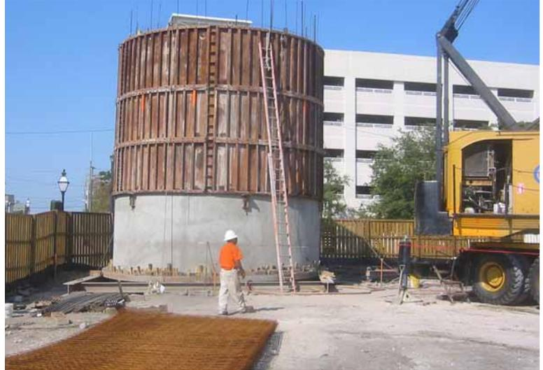
Construction of the tunnel shaft at Plum Island will look similar to this shaft construction on Calhoun Street, which was part of the Cooper Sewer Tunnel Replacement Project (2007). The Plum Island shaft will be 130 feet deep. It will provide access for tunnel construction and will be turned into a new pump station when the tunnel is complete.
