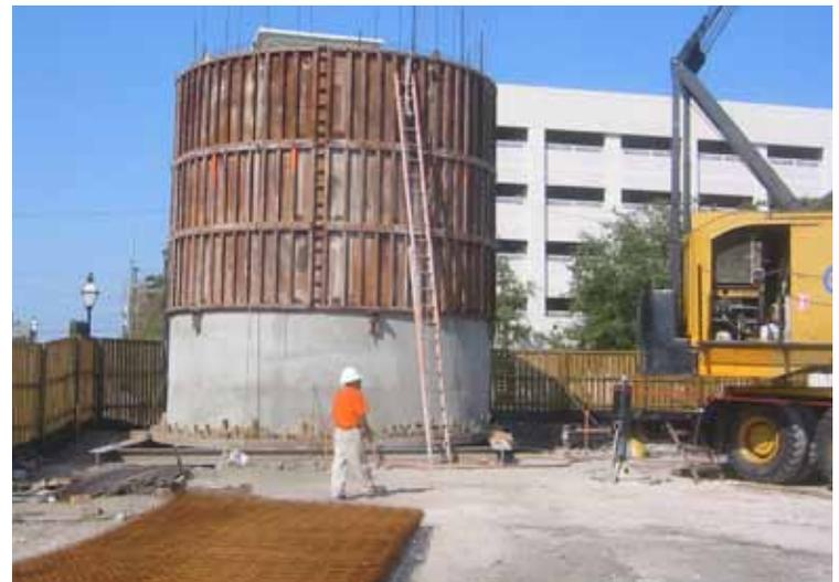
Work activity at the Croghan Shaft site will look similar to this drop shaft construction on Calhoun Street, which was part of the Cooper Sewer Tunnel Replacement Project (2007).
